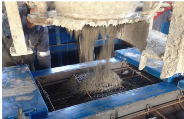
**Figure 1. Dumping of the concrete in the mould**
