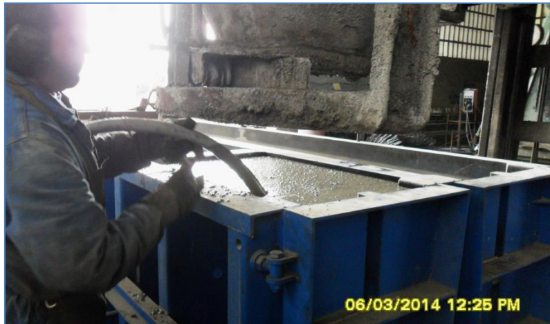
Compacting process through vibrator needle
