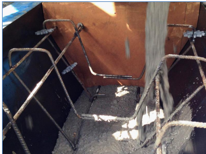
Dumping of the concrete in the mould
