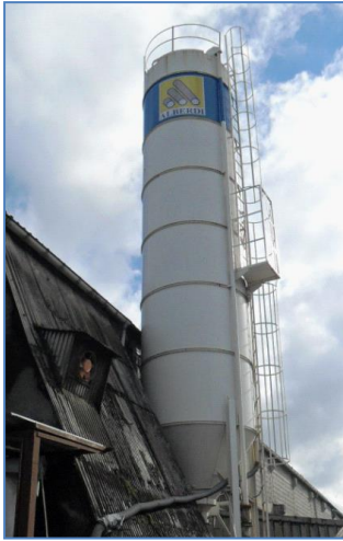
Cement storage silo
