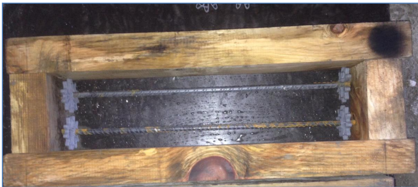
Image of a mould to manufacture a barrier with reinforcement
